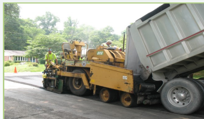
Typical hot mix asphalt paving operation
